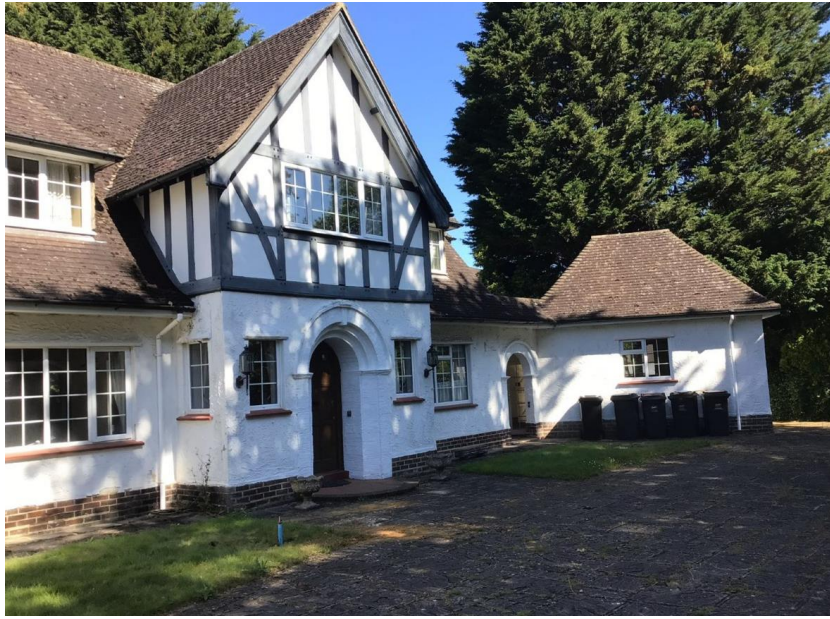
Figure 4: Front of existing dwelling including single storey element
